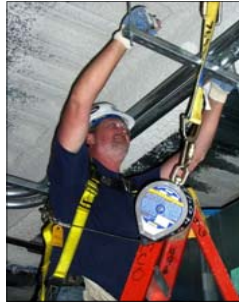
Tim Kelton hanging a unistrut rack.
