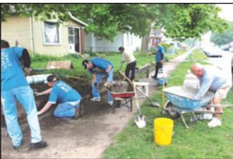
ERMCO volunteers build retaining wall at Rebuilding Together 2010
